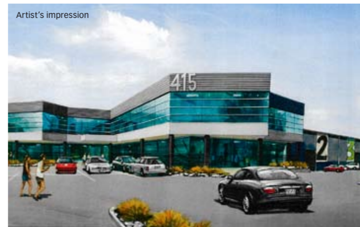
Building repositioning underway at 415 Church St, Penrose
