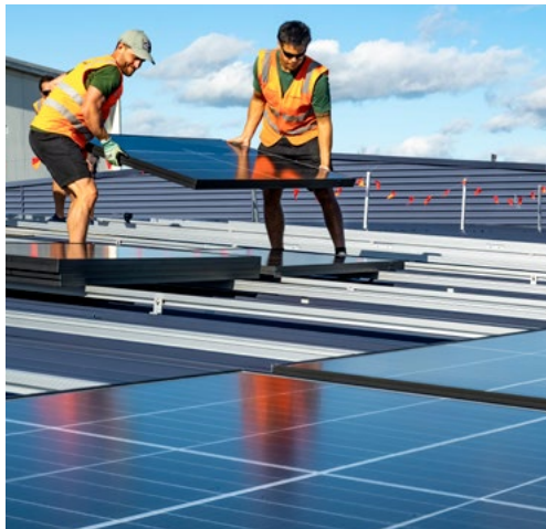
– Solar installation at 3-5 Niall Burgess Road.
